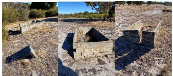
3 x brick and concrete horse troughs
